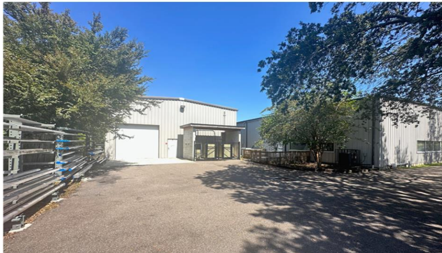
Exterior view of warehouse #2 looking N.
