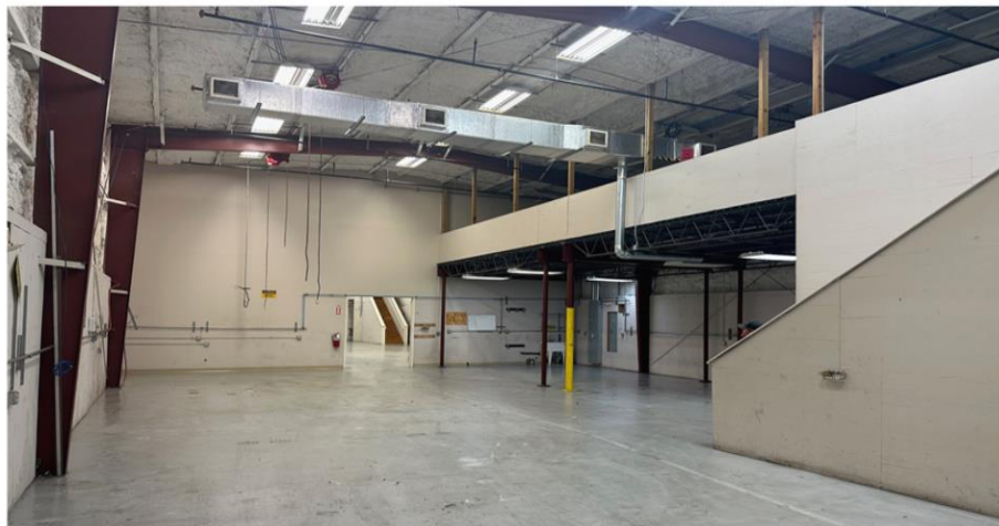
Interior view of warehouse #2
