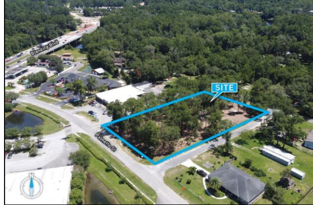
Aerial view of subject looking north
