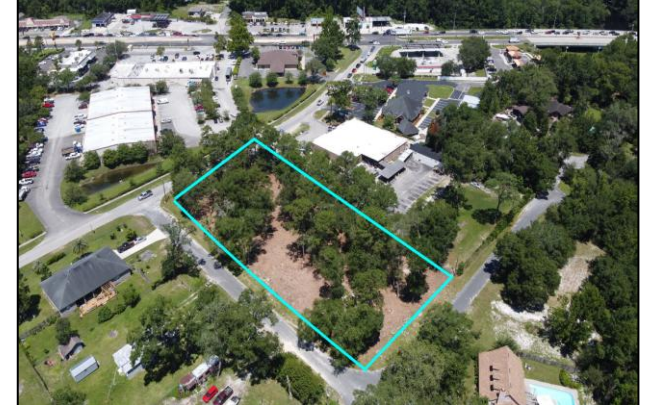
Aerial view of subject looking west
