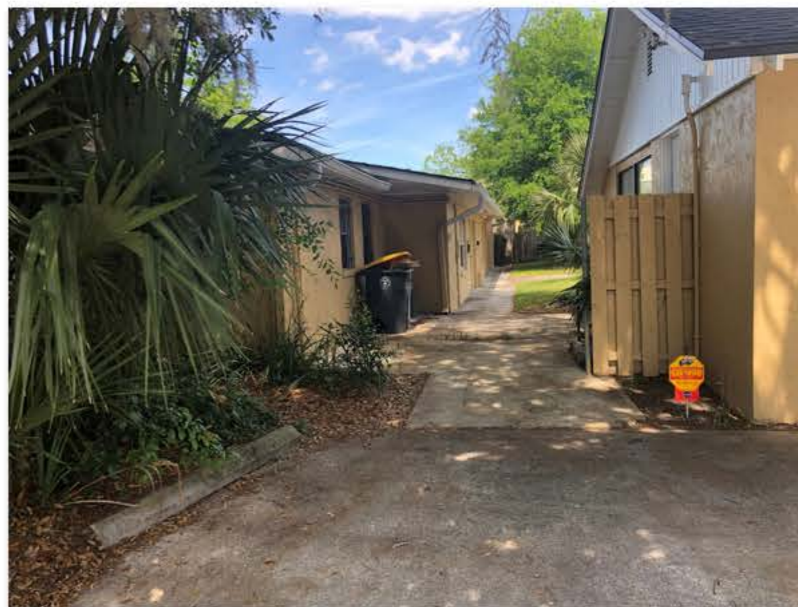
View of building 2 -1914 Art Museum suites B-D
